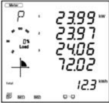
Figure 3-7 - Three-Phase Power Page
