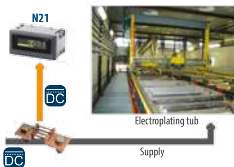
Current measurement in an electroplating plant
